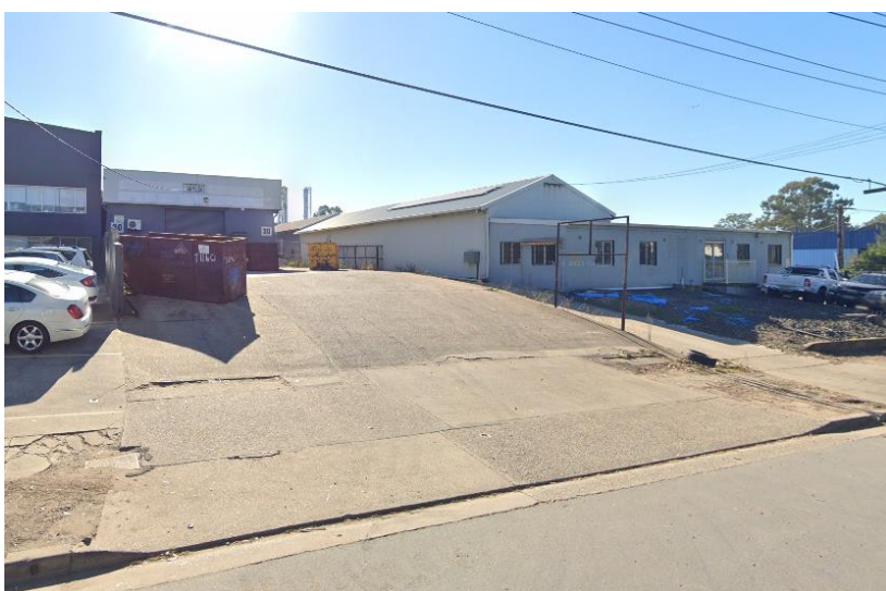
Figure 3 Tattersall Road frontage
